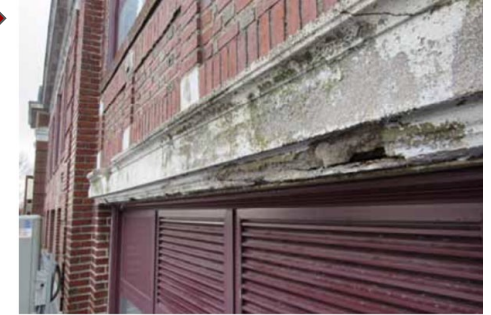
View of pronounced stone cladding deterioration as seen at north facing elevation of original building—also note exposed and corroded reinforcing steel
